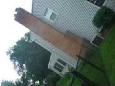
1 Excessive spalling
